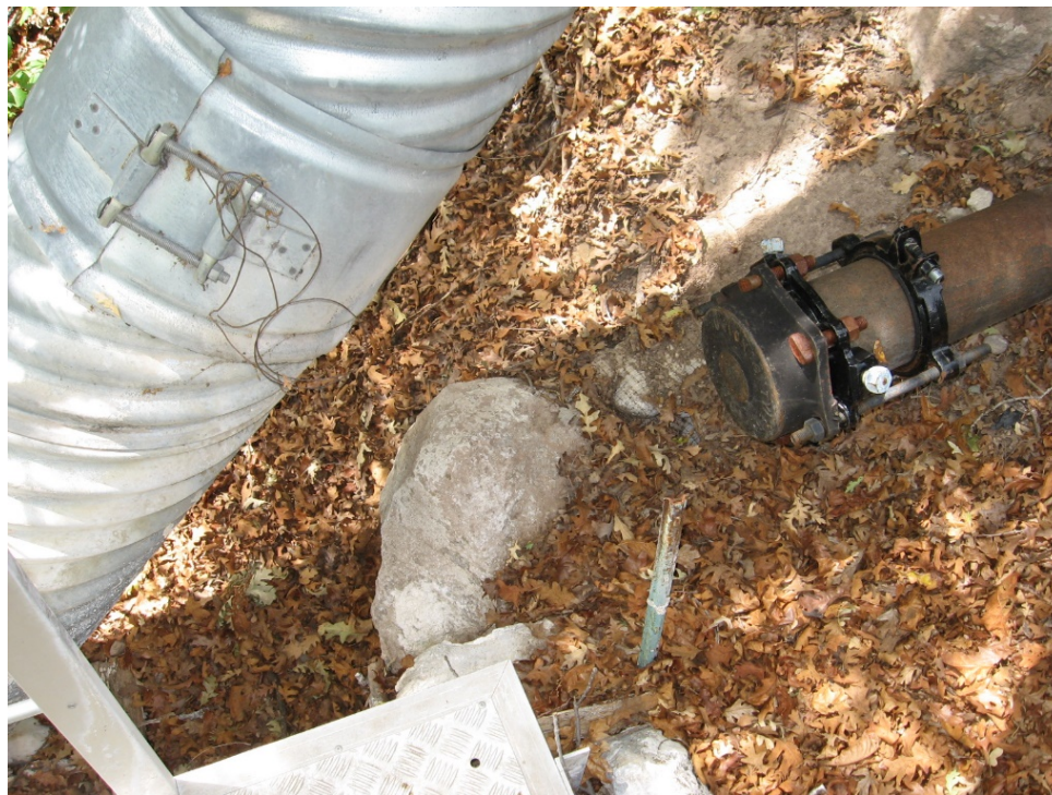
Photograph - NPDES-03A027-18-002 Outfall 03A027 Condition at Discharge Location
